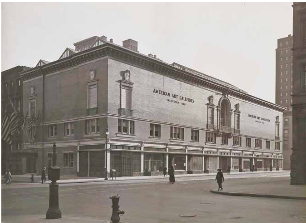
Figure 8: This building, which filled the east side of Madison Avenue from East 56th Street to East 57th Street in New York City (the view here is south down Madison), twice briefly housed the manuscript of “ The King of the Foxes ” – during its first public sale in 1923 (by the American Art Association) and during its third public sale in 1945 (by Parke-Bernet Galleries). John Wallace Gillies, “American Art Association Building in New York City, 1922” (Smithsonian Institution, Archives of American Art, American Art Association Records).
